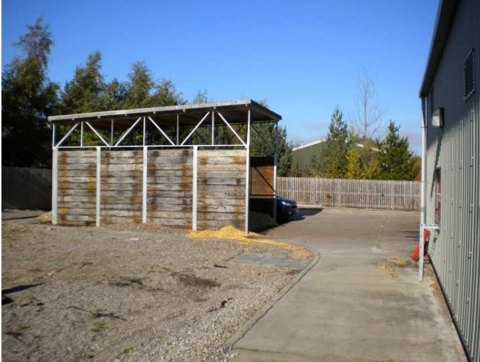
Additional fuel storage
