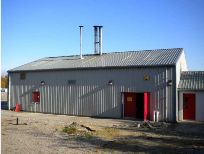
Boiler house with fuel storage
