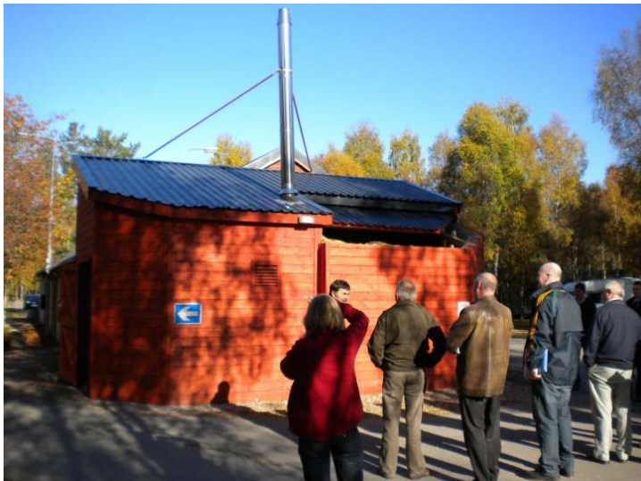
Caravan boiler house with storage
